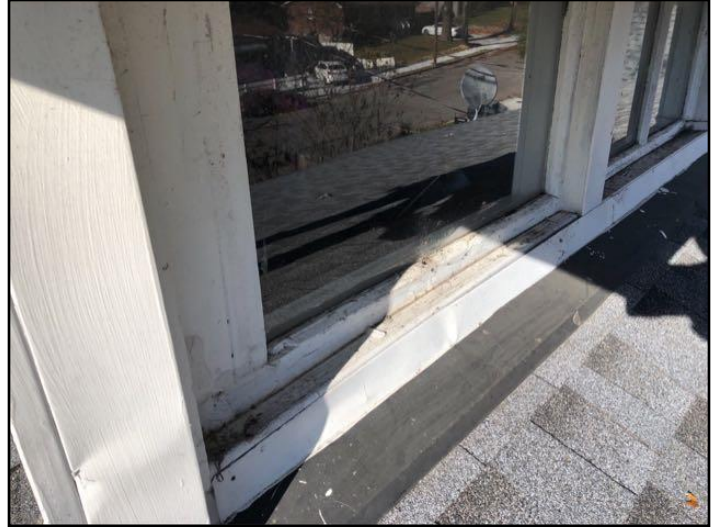
3. Loose, damaged, patched, open seams
