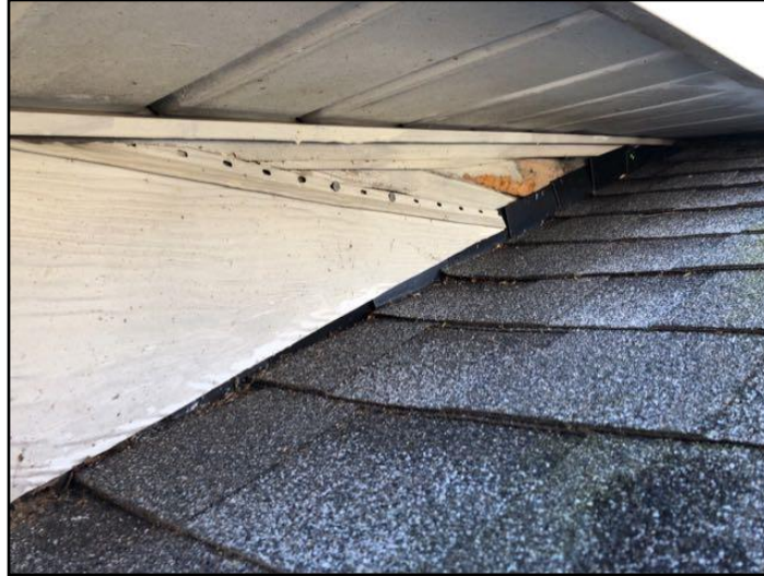
14. Flashings incomplete or ineffective
