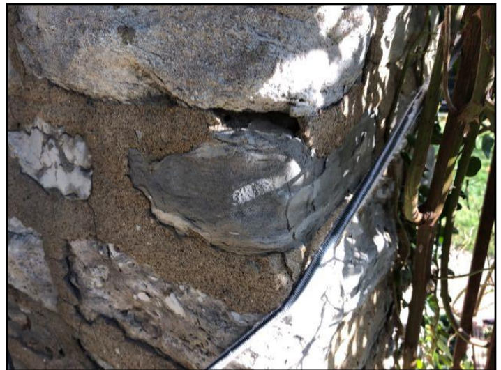
23. Mortar deterioration
