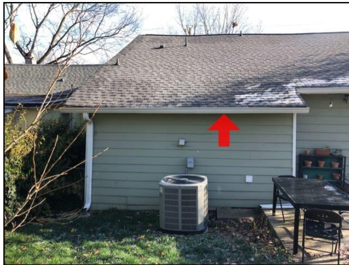
7. Improper slope, ponding
