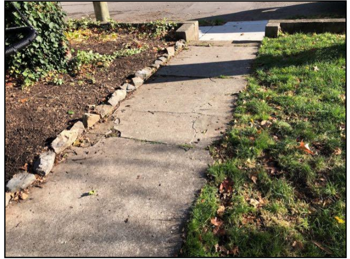
39. Cracked or damaged surfaces
