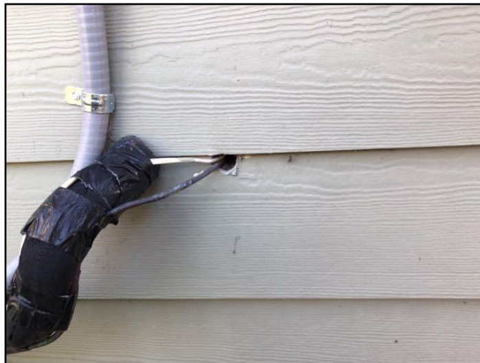
25. Unsealed Openings in Siding
