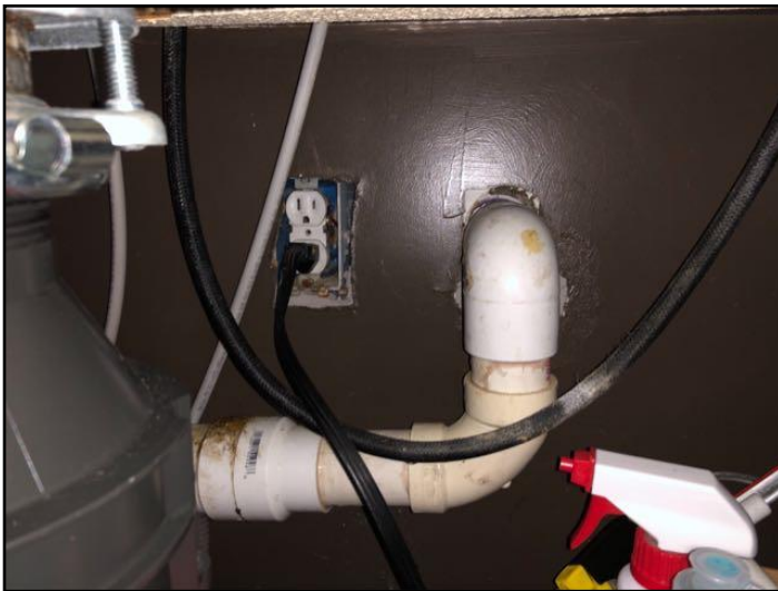
129. Unsealed openings for plumbing penetrations
