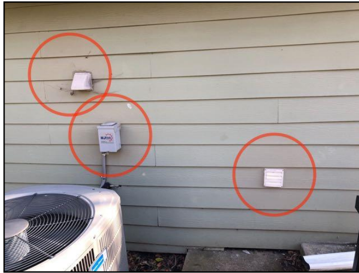
27. Missing Plinth or Mounting Block
