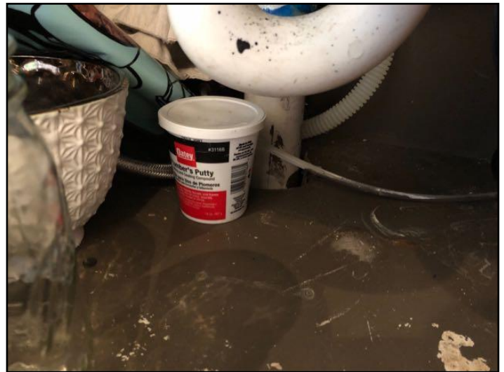
130. Unsealed openings for plumbing penetrations
