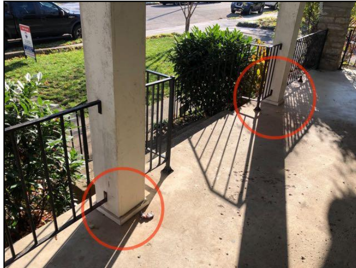
31. Column in Contact with Concrete
