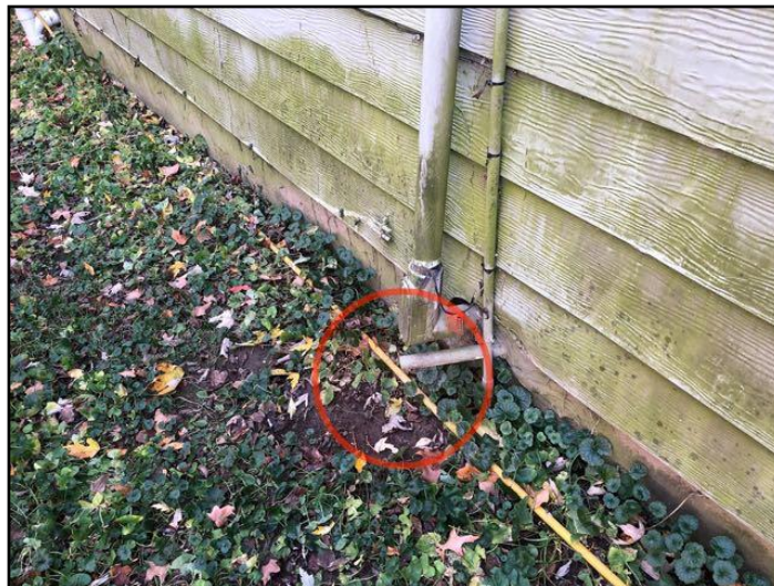
82. Improper discharge point
