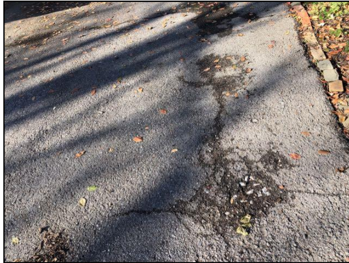
41. Cracked or damaged surfaces
