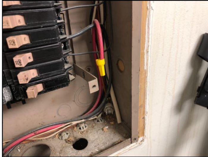
74. Abandoned wires in panel
