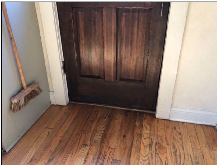
126. Weatherstripping missing or ineffective
