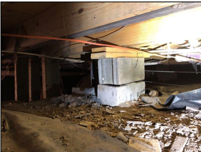
51. Improper shim and installation
