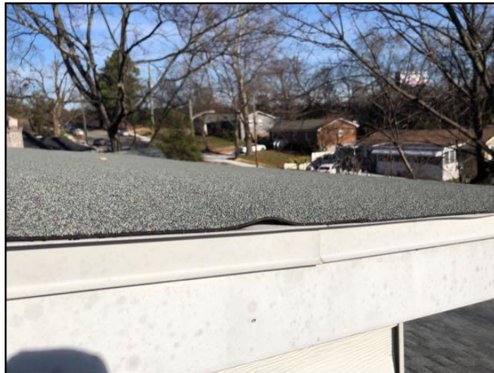
5. Openings at seams or flashings
