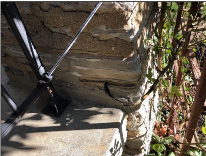
22. Mortar deterioration
