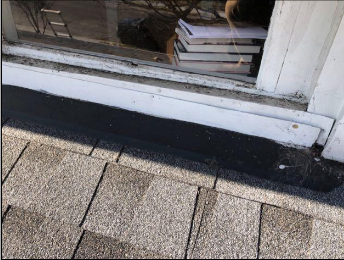
2. Loose, damaged, patched, open seams
