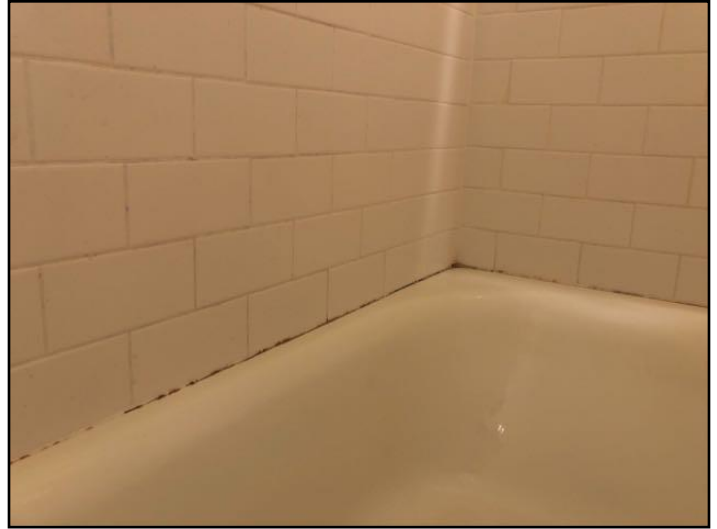
103. Caulking loose, missing or deteriorated
