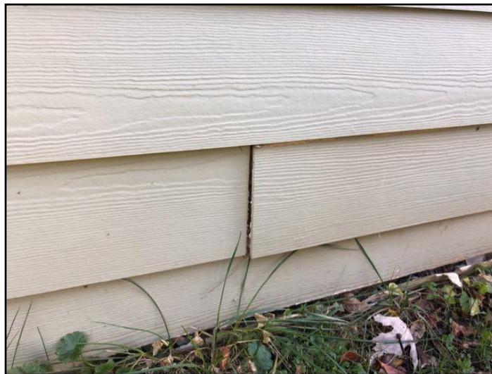
26. Missing Caulking (or Back Flashing) at...
