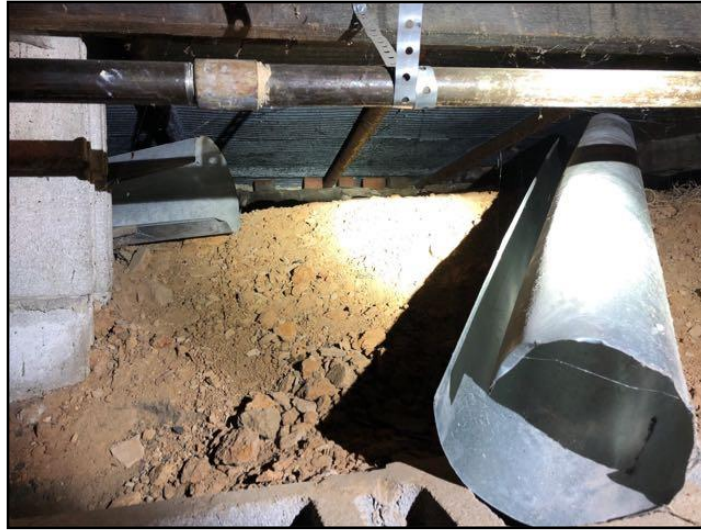
89. Incomplete vapor barrier
