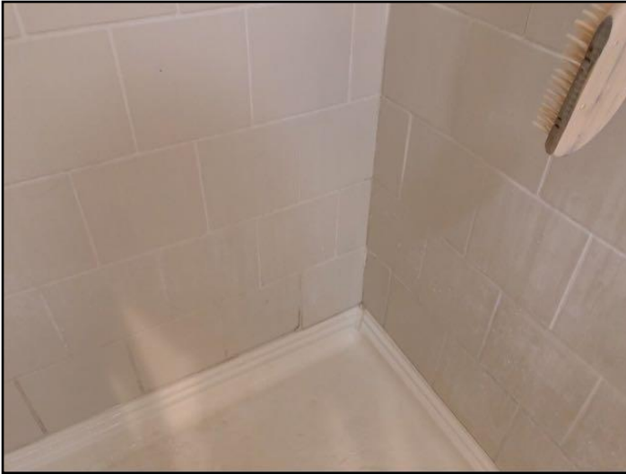
108. Grout loose, missing or deteriorated
