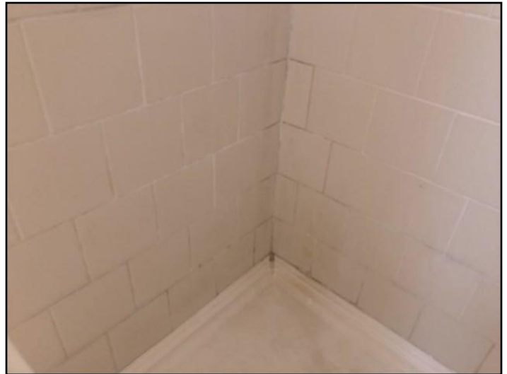
107. Grout loose, missing or deteriorated
