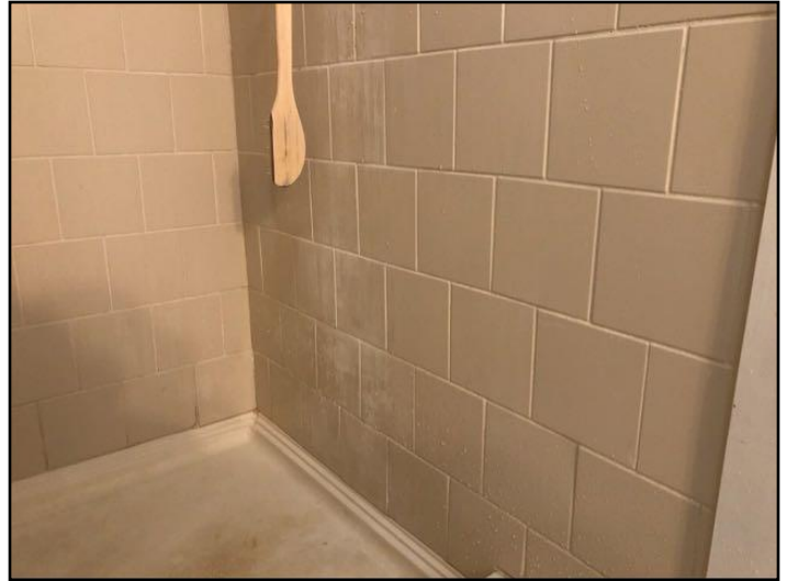
109. Grout loose, missing or deteriorated
