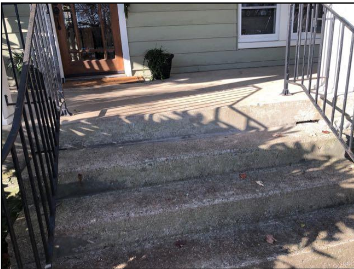
32. Steps or landings settling or heaving
