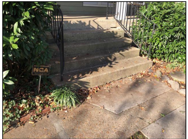
33. Steps or landings settling or heaving
