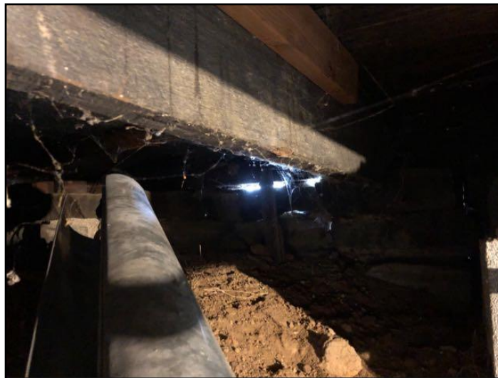
48. Holes in Foundation Wall
