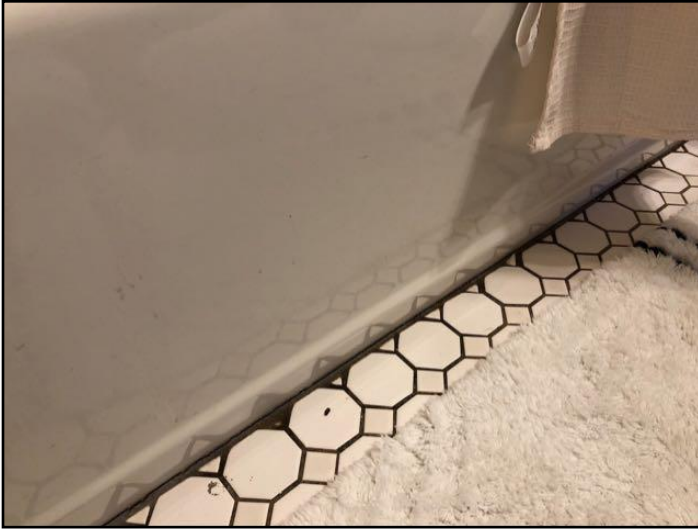
102. Caulking loose, missing or deteriorated
