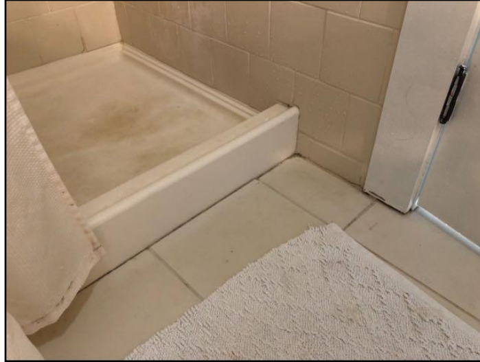
105. Caulking loose, missing or deteriorated
