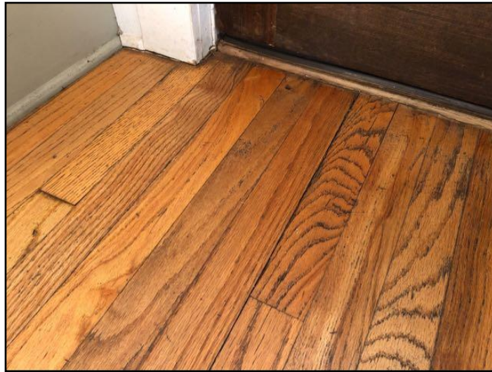
114. Wide seams between floorboards
